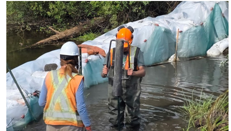
COFFER DAM AND POST DRIVING, BLACKWATER
